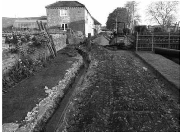
Work started in April and a trench was dug across the kitchen garden, under the stream and then through the yard to the boiler room. Work was severely hampered by torrential rain which caused the sides of the trench to fall in but the devastation was cleared up before the first open day in May and the system was up and running very soon thereafter.
